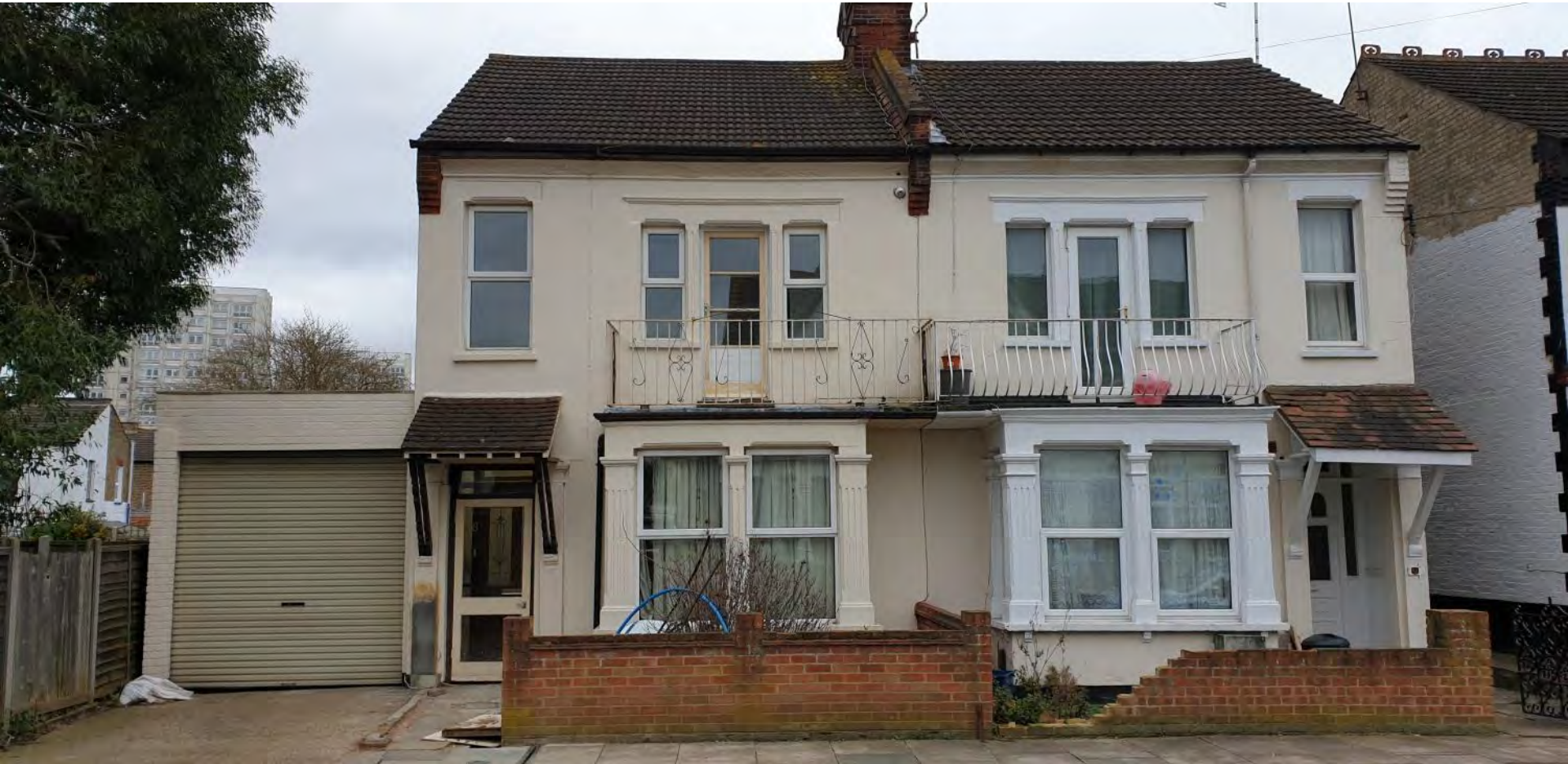
Front elevation during refurbishment, 2019
