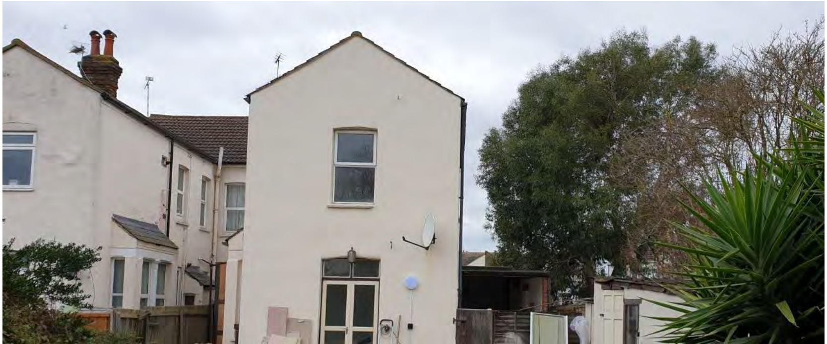
Rear elevation of site during refurbishment in 2019
